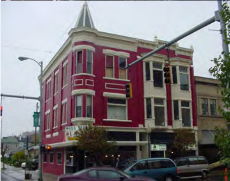
Before and after renovation of local restaurant, Toro Loco.
