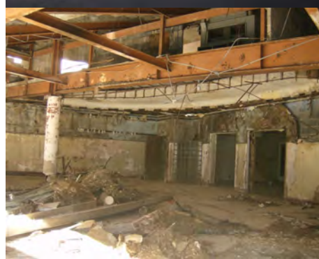
Ro-Na Theater Renovation Project
